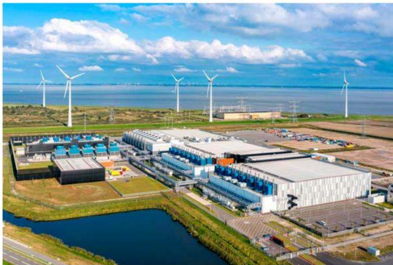
Figure 6.8 The Google data center facility in Eemshaven, Netherlands. In addition to the multiple, multistory buildings that host the IT equipment in racks, the picture shows the transformers, switchgear, and generators needed to operate a WSC.
